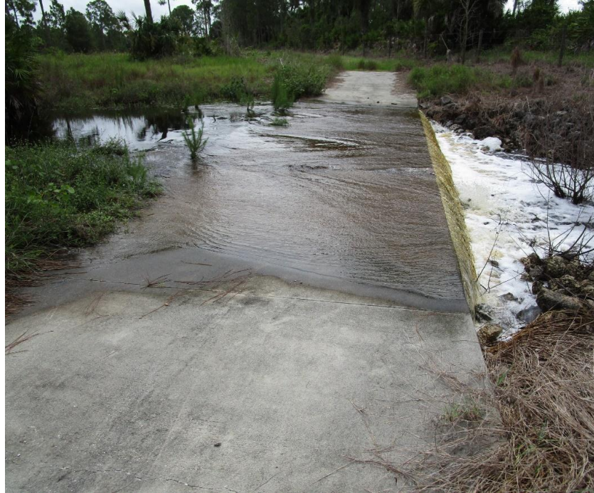
Figure 3-17. Concrete Low-water ford in South Yucca Pens
